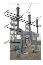
HV sensor system providing monitoring and fault detection and diagnosis technology to provide a trip signal to a switching or protection device
